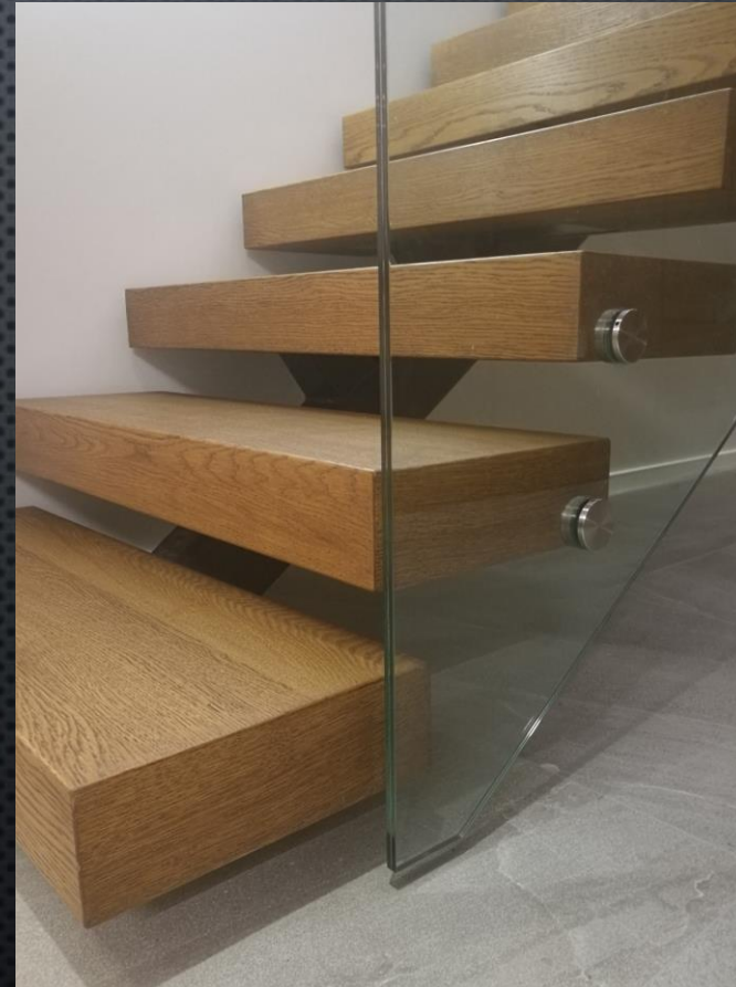
Massive wooden steps, metal beam of stair
